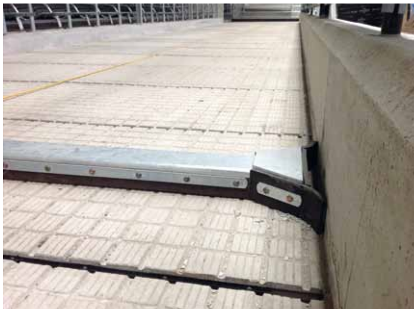
• Slatted floor scraper with trapezium end
