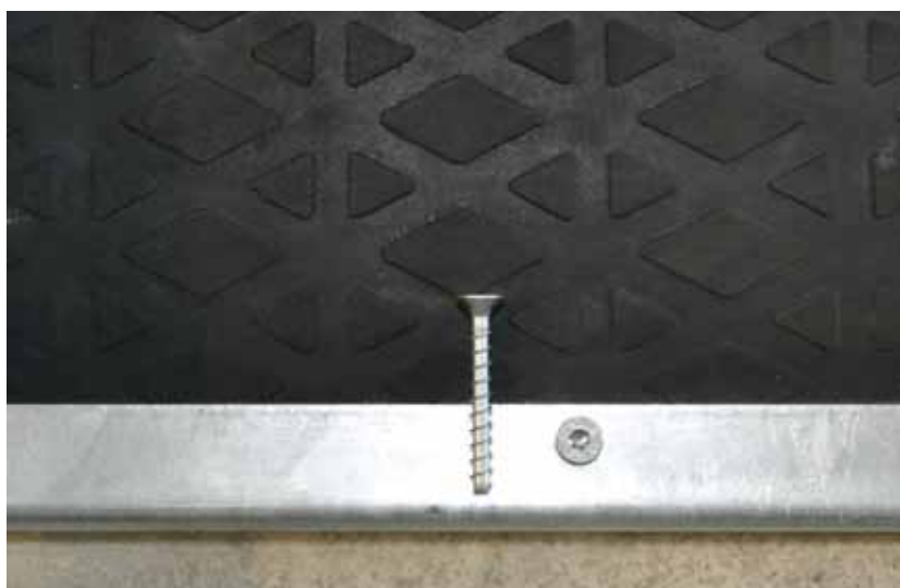
• Galvanized fastening profiles are installed with concrete screws
